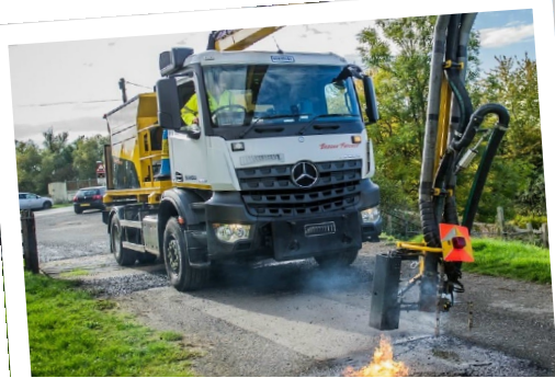
Above: The Dragon Patchers can fix more than 1,000 potholes every week
